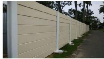
Pre-Cast Steel Reinforced Concrete Wall (Principle 40)
